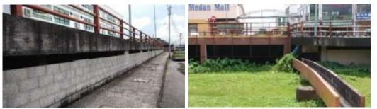
(b) No wall at inaccessible places (a) Concrete block wall along pedestrian path Figure 6: Public accessibility control underneath the platform
