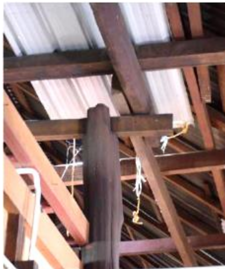
Figure 3. Melanau Tall Longhouse Mortise and Tenon Jointing between Column and Beam.
