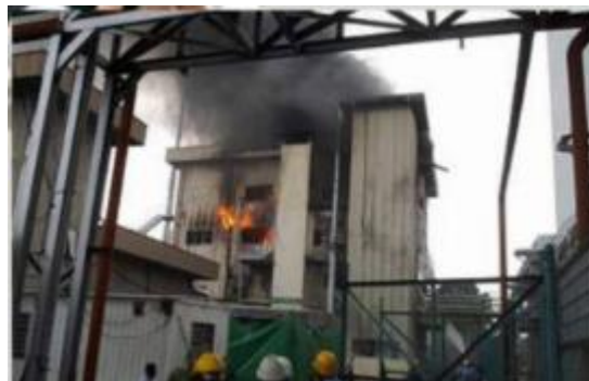
Figure 6. Factory in Seberang Jaya, March 2013
