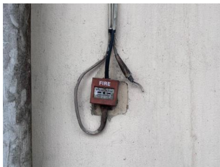
Figure 5. Damaged fire equipment (fire break glass)
