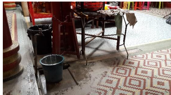
Figure 8. Scupper drain along perimeter of Inner Courtyard. (Source: Author, 2017)
