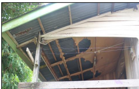
Figure 13: Poor Quality materials and Lack maintenance
