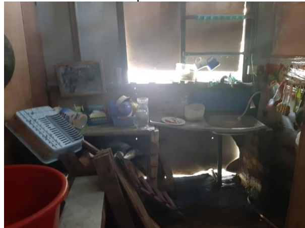
Figure 9: Internal condition of Respondent F house
