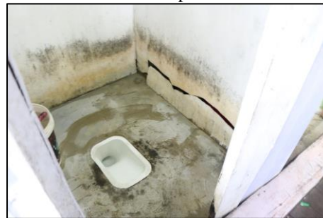
Figure 17: Internal settlement problem
