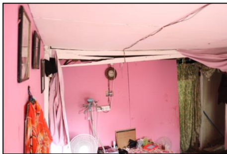
Figure 17: Internal settlement problem
